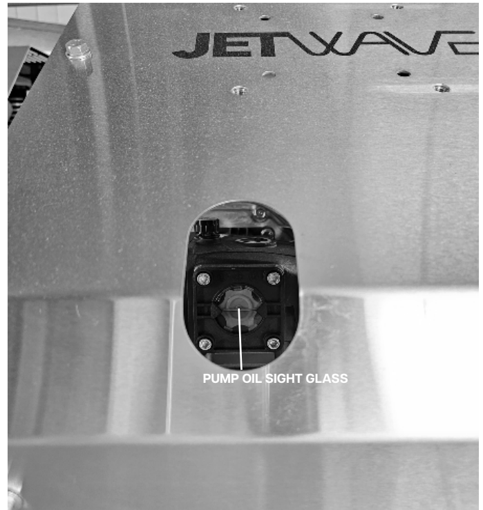
Figure.10 - Checking Pump Oil Level
